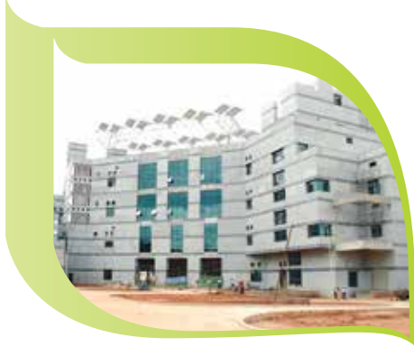
Instem building - NCBS campus
