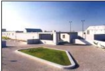
Gujarat Powergen Energy, Paguthan /Bharuch
