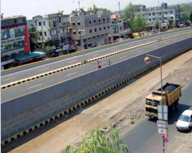
Pimpri Chinchvad Flyover Project
