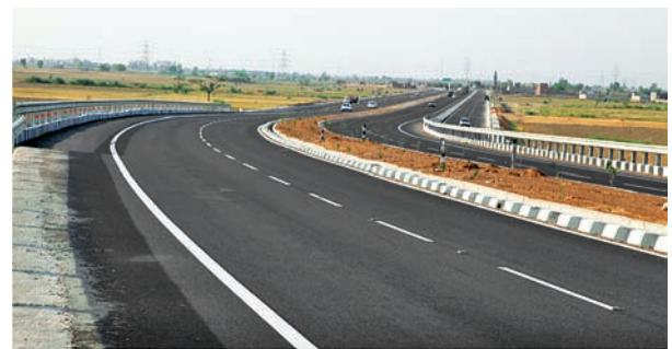
Rohtak-Bawal Road Project
