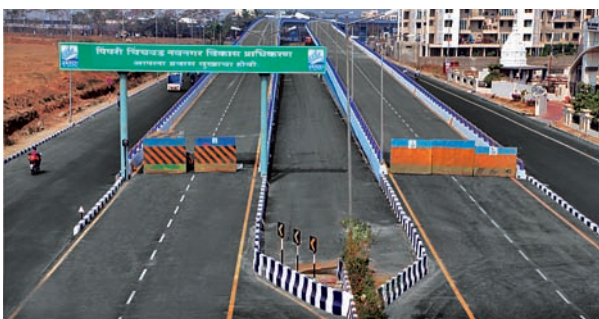
Fly Over and Elevated Road, Mumbai - Pune National Highway
