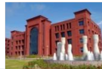
Syntel International, Pune
