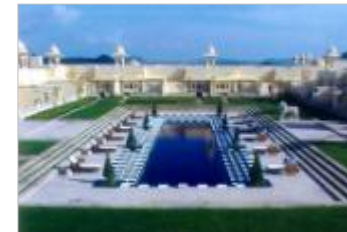
Udaivillas/Oberoi Hotels, Udaipur
