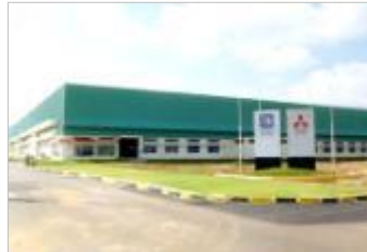
Hindustan Motors, Chennai
