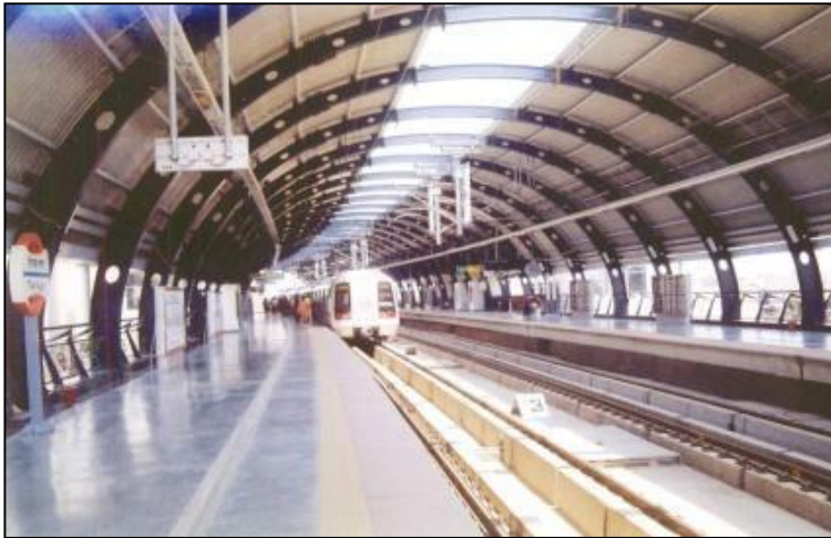
Elevated Metro Stations, DMRC, Delhi
