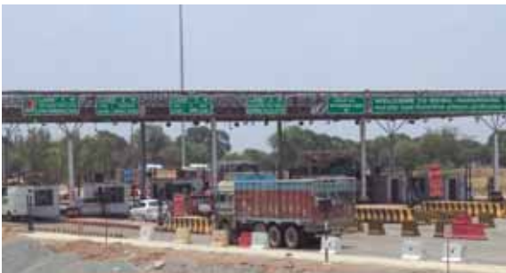
Rewa Hanumana Road Project Toll Plaza 2
