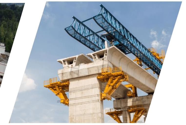
Urban Infra & Metro Rail
