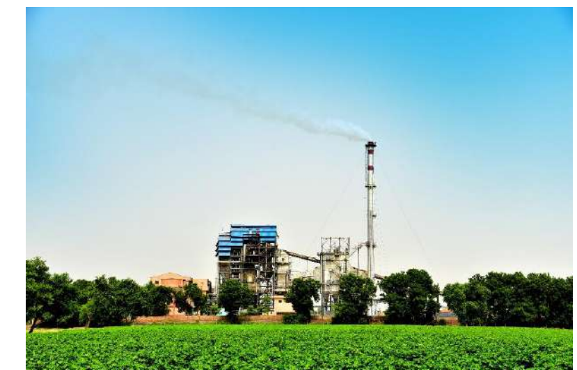
Padampur Power Plant, Rajasthan (India)
