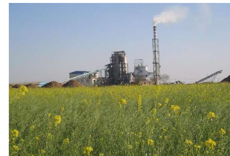
Uniara Power Plant, Rajasthan (India)
