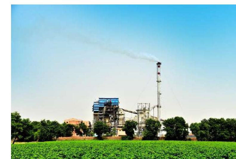
Padampur Power Plant, Rajasthan (India)
