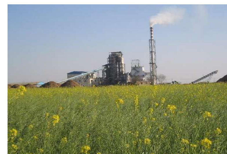
Uniara Power Plant, Rajasthan (India)
