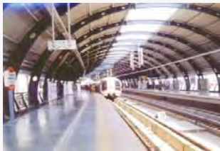
Elevated Metro Stations, DMRC, Delhi
