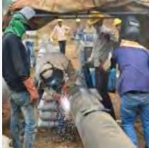
Thumbli Water Pipeline– Cairn Energy India – Rajasthan
