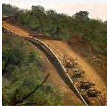
Panvel Dabhol Pipeline Project–Gail Ltd - Maharashtra
