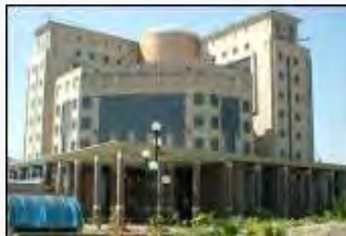
Power Grid Corpn., Gurgaon
