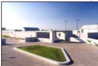
Gujarat Powergen Energy, Paguthan /Bharuch
